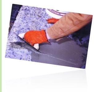
Ez PATCH is packaged as a three component system in a single pail. Removing the lid you will see a cradle holding Part B of the two part 100% resin epoxy. After removing this cradle you will note that the rest of the pail contains Part A mixed with a special aggregate. You simply open Part B and pour it into this admixture and mix thoroughly to fill your holes, joints, cracks and damaged areas. Thats it! No measuring and no mistakes.
